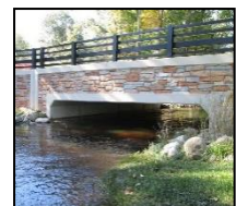
Figure 4: Three-sided box bridge
