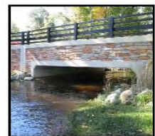
Figure 4: Three-sided box bridge
