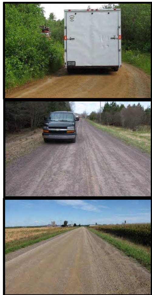
Figure 2: Top – Road with IBR number of 1 road that has poor surface width, poor drainage adequacy, and poor structural adequacy. Middle – Road IBR number of 7 that has fair surface width, fair drainage adequacy, and fair structural adequacy. Bottom – Road with IBR number of 9 road that has good surface width, good drainage adequacy, and good structural adequacy.
